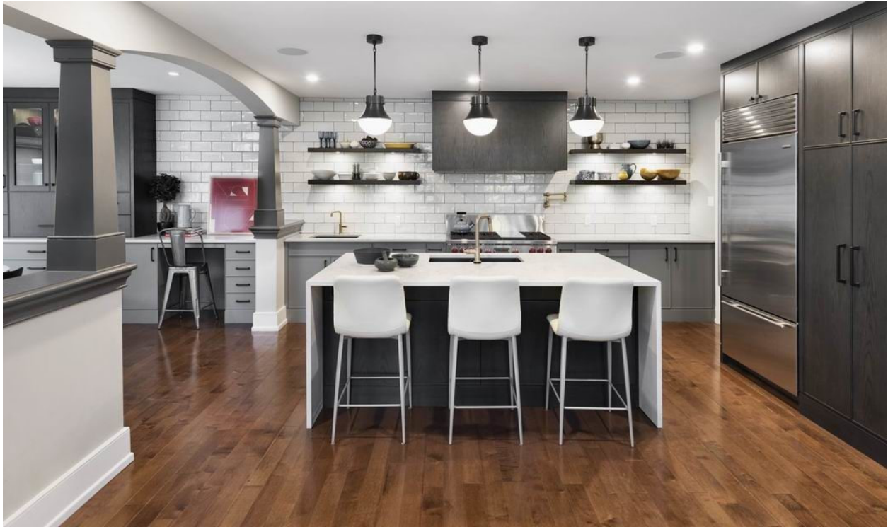
The cabinetry in this project had to be reconfigured when a hidden structural beam was discovered during demolition. Photo courtesy Amsted Design-Build / StyleHaus Interiors / Irpinia Kitchens
